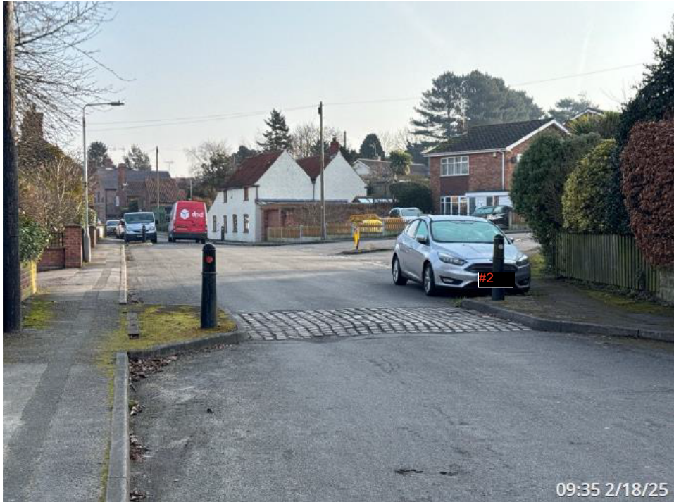
Figure 6 - Speed hump condition 2, Station Rd
