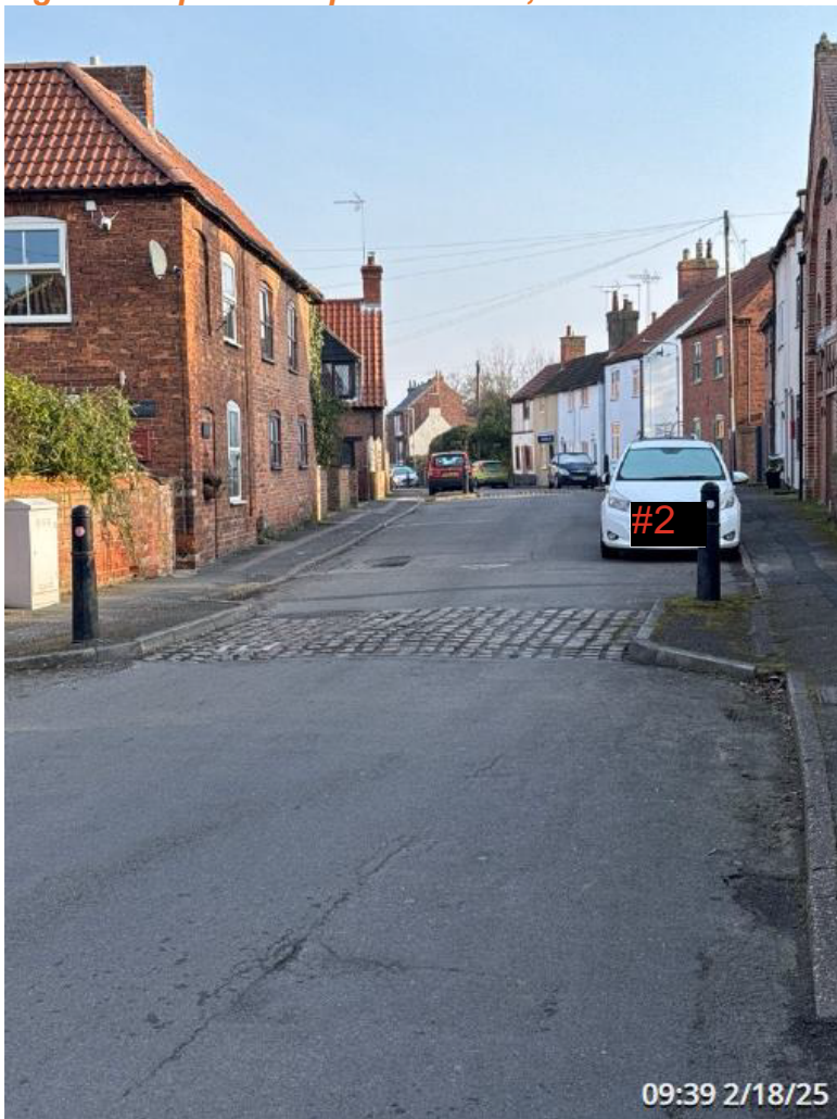
Figure 7 - Speed hump condition 3, Station Rd
